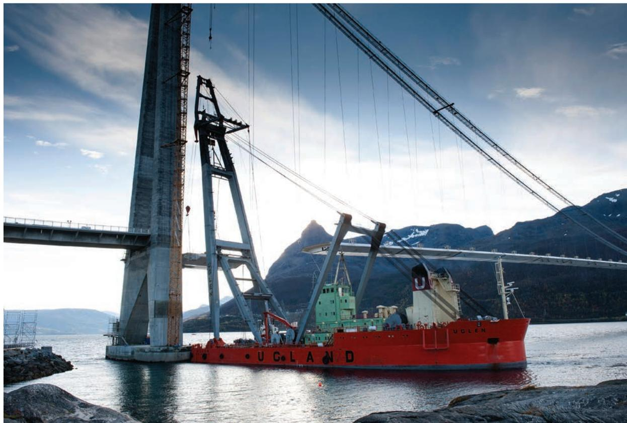
HLV Uglen installing bridge elements at the Hålogaland bridge in northern Norway
