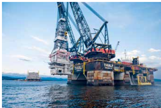
Coupling You can see here the drilling module from Nymo in Grimstad in the lifting gear, as previously described, ready to be hoisted onto the platform by Thialf in Klosterfjorden, north of Haugesund
